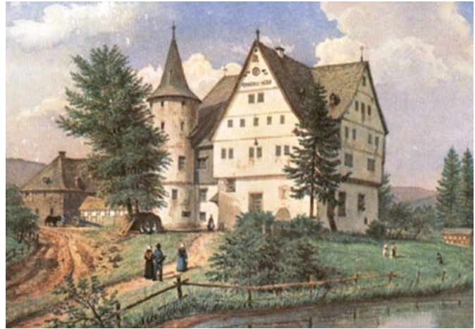
Fig. 3. Junkerhees Castle in the 1700's. The bottom section has 2 meter thick walls and was built for defense by the knight Adam von der Hees in 1523. The decorative upper floors were added in 1698. 7
