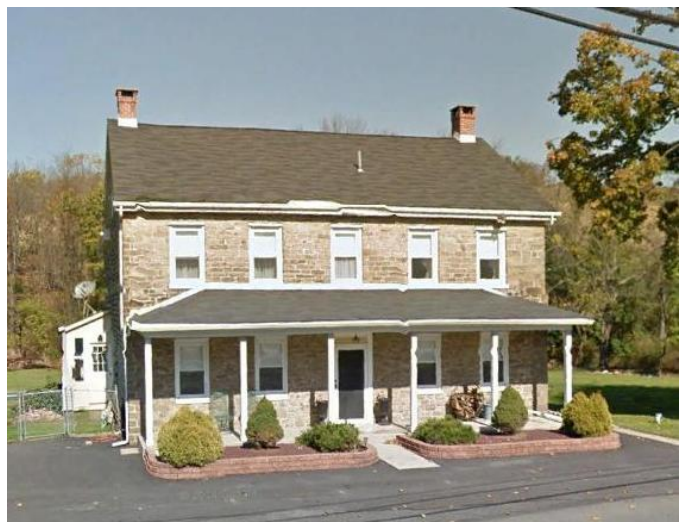
Fig. 3. Old house stands on land once owned by Peter Anthony and approximately at the site of Anthony’s Tavern. The history of this building is unknown to the author. Google Earth Street view image.
