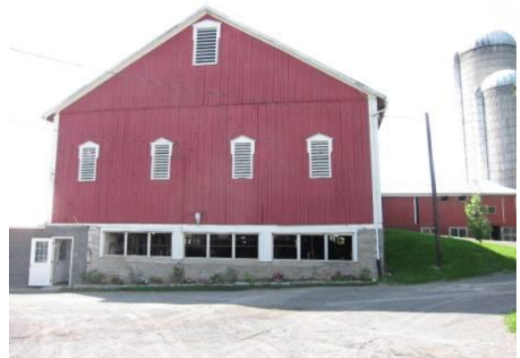
Fig. 11. Side view of the barn as it appears today. It was built in the late 1700's, possibly by Martin Dreisbach Jr.
